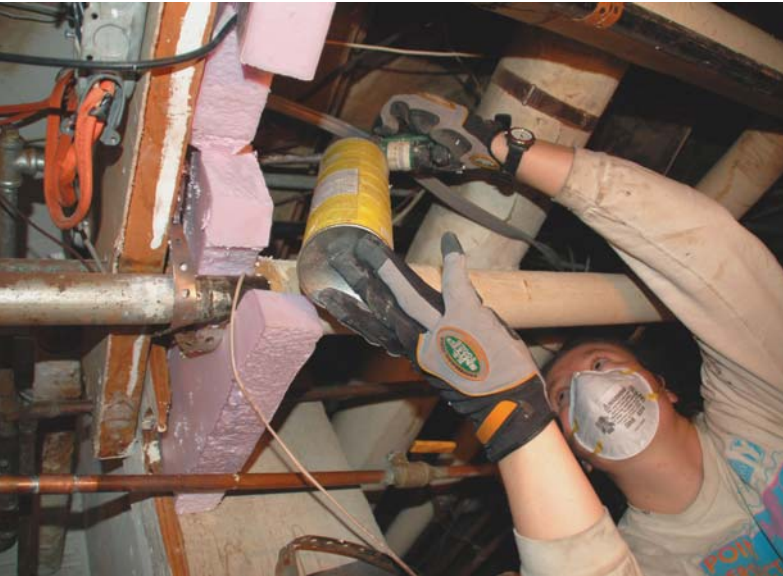
Lexie Hain works to create an airtight closure for an above-grade crawlspace.
