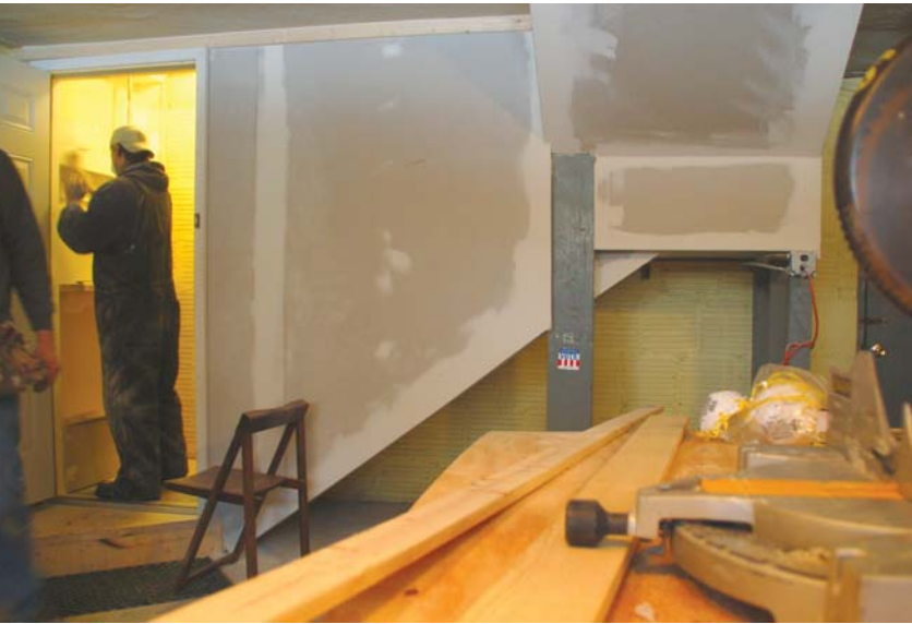
Jason Whitmarsh puts the final touches on a recently enclosed stairway, once a massive chase between unconditioned and conditioned space.
